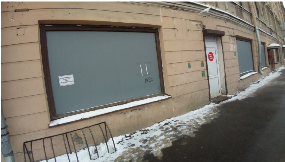
Fig. 1. A dark store in a former regular store, St. Petersburg, February 2021. Photo by K. E. Axenov
